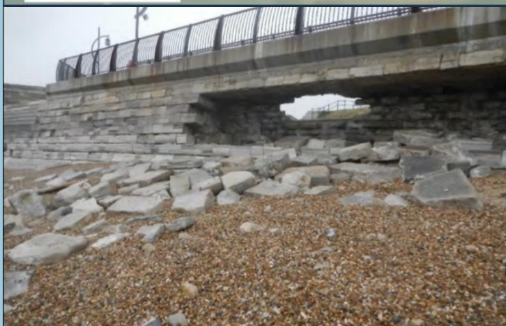
Long Curtain Moat - Feb 2014
