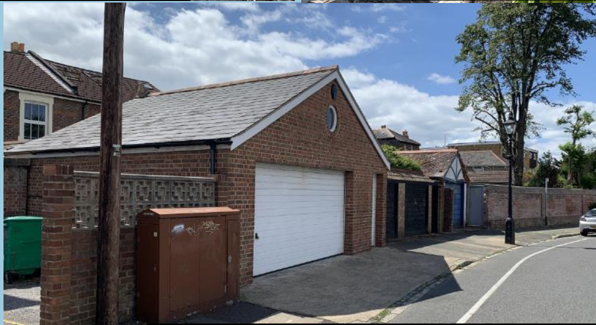
Similar garages along St Bartholomew's www.portsmouth.gov.uk
